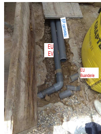
EVACUATION EP - Diam. 160 mm
